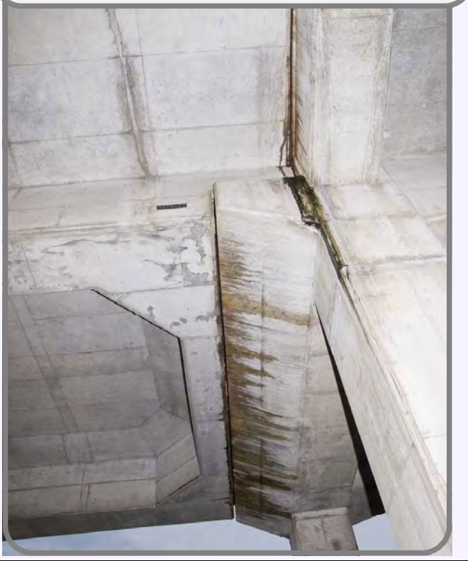
Fig. 2. Photo of the Joetsu Shinkansen railway showing the crevices.
